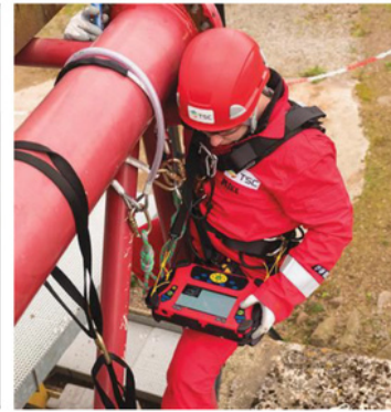
Figure 9. Rope-access inspection with ACFM
